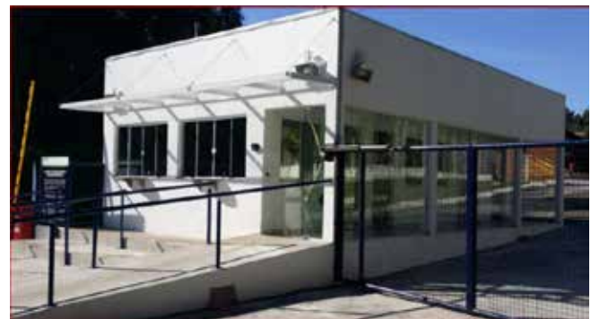
Figure 7. Access to the company after implementation of improvements
