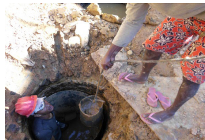
Figure 5.6. Cargo transportation - pipe cleaning
