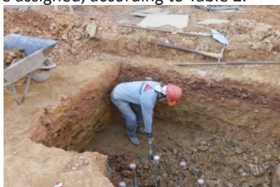
Figure 5.1. Excavation of blocks
