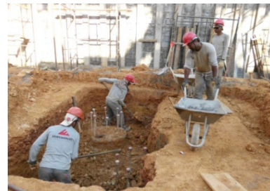
Figure 5.5. Cargo transportation - excavation
